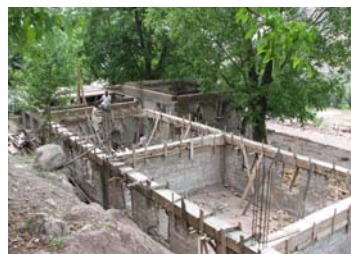
Work in progress on the first academic block
