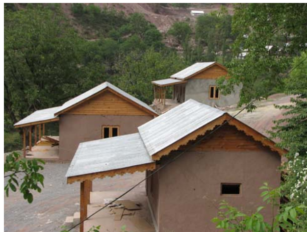
Temporary classrooms nearing completion
